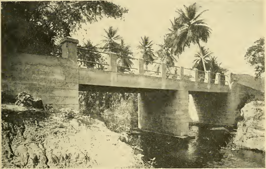
A TYPICAL CONCRETE BRIDGE ON THE PUERTO CABELLO-VALENCIA ROAD
